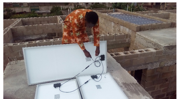
Figure 4: The solar panels being fixed
